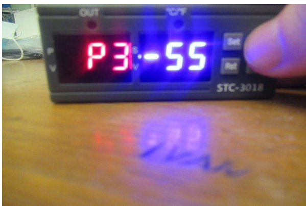
Low temperature alarm
